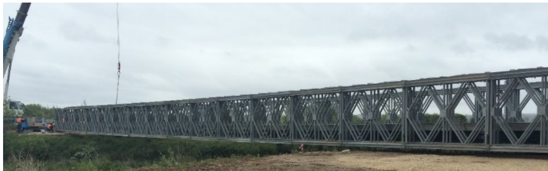
Fig. 2. Bailey bridge for route reestablishment during the collapse of a section of Highway A14 – Figueira da Foz/ Coimbra, Portugal (2016);
